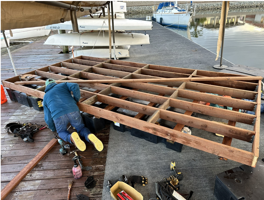
Staff hard at it building sample Dock section.
